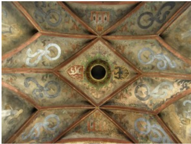
The net vault of the Old Town Bridge Tower.
